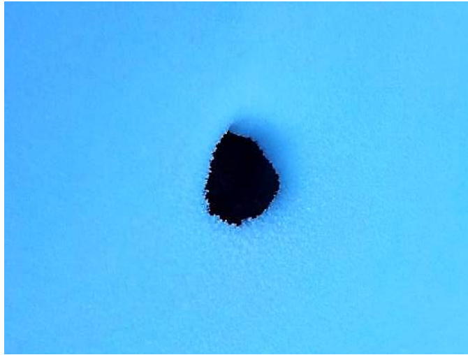
Figure 2: Roof Drain Clear of Ice Build-up.
