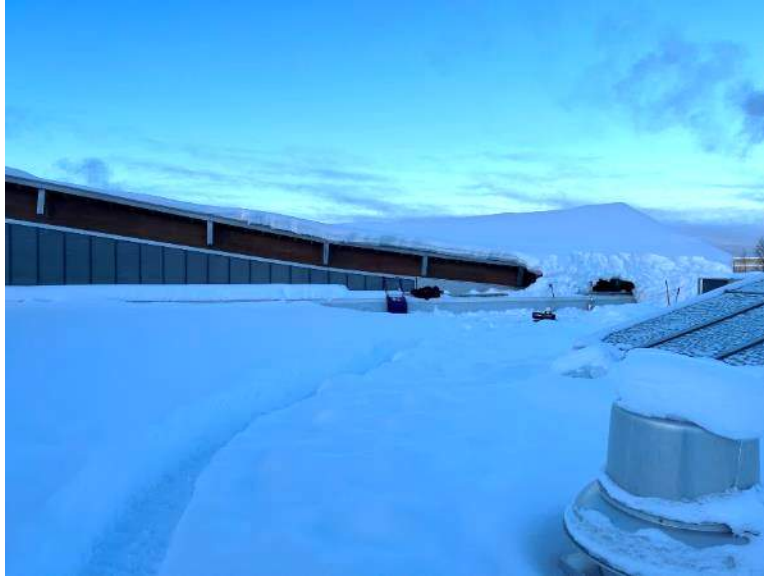
Figure 4: Sliding snow at Location #5.
