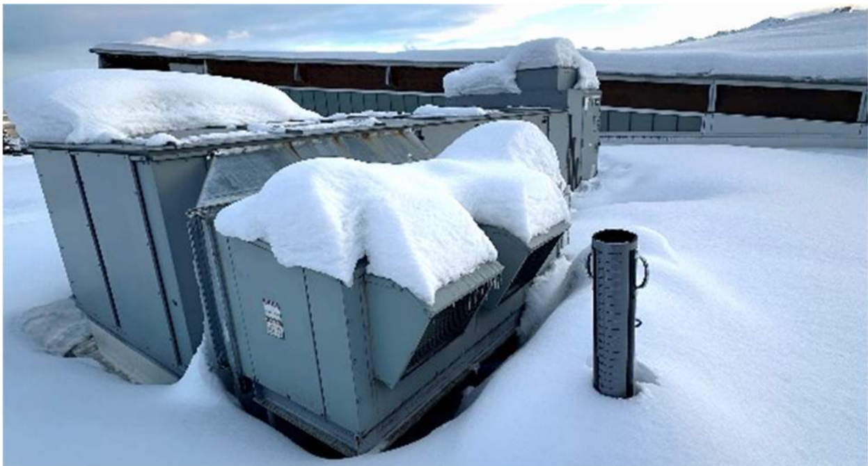
Image 1: Drifting Snow at RTU (location #3).
