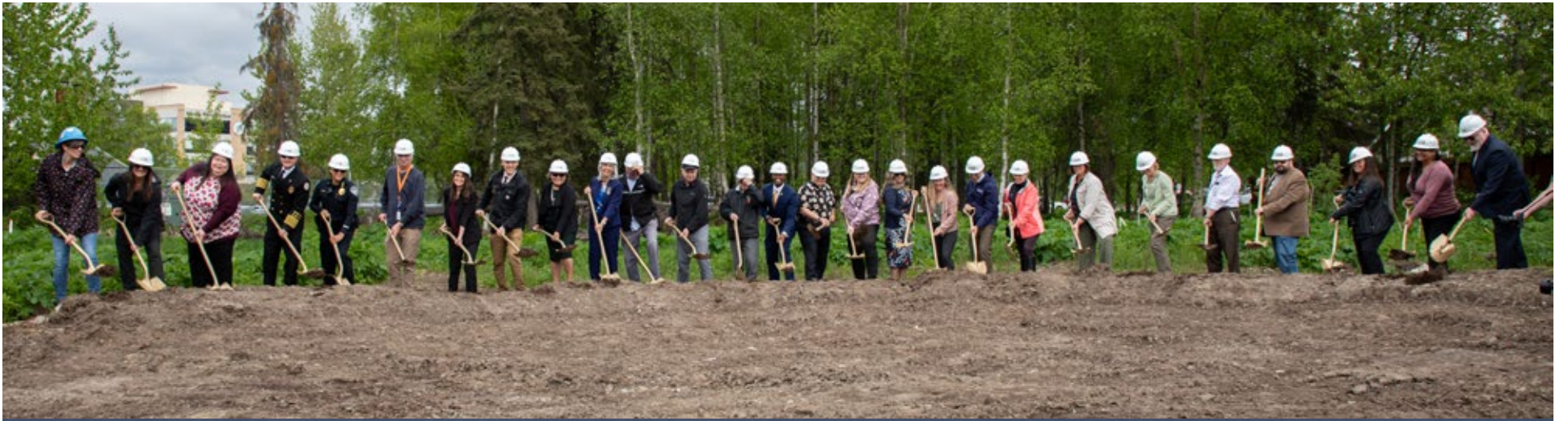
Southcentral Foundation hosted a groundbreaking on a behavioral health expansion project in Anchorage with federal, state, and local dignitaries along with community partners.
